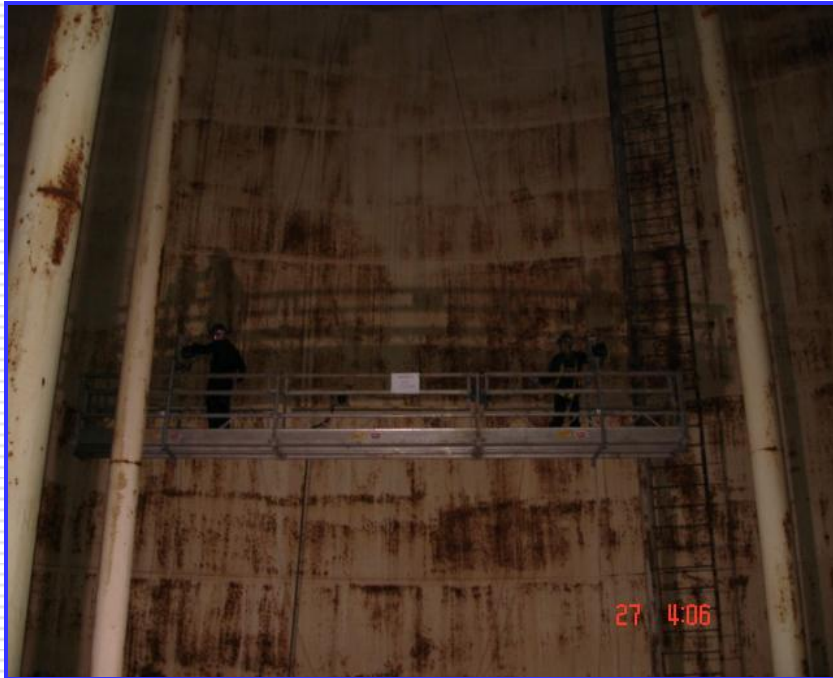
Movement of Spreader System Gondola on Tank Shell
