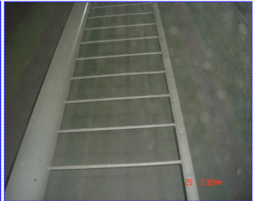
Complete Painting of Tank Ladder Internal
