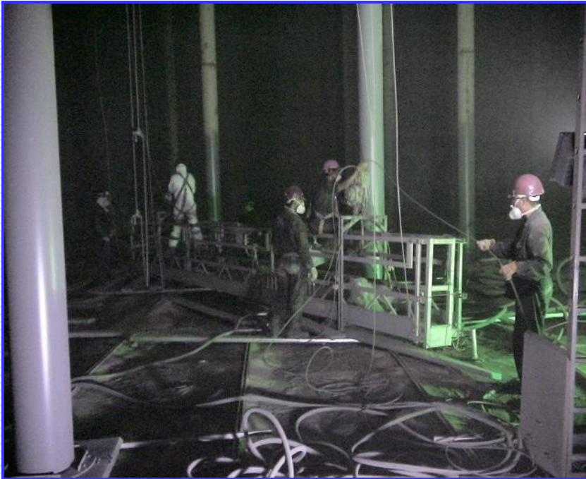
Movement of Spreader System Gondola to the next location
