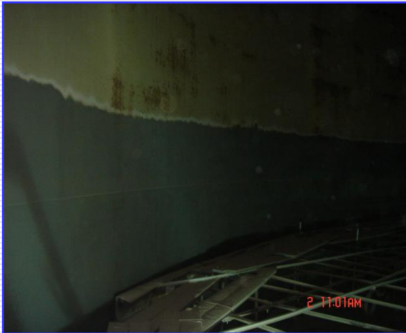
Blasting of Tank Shell
