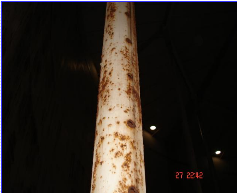
Before Blasting and Painting of Tank Column Internal
