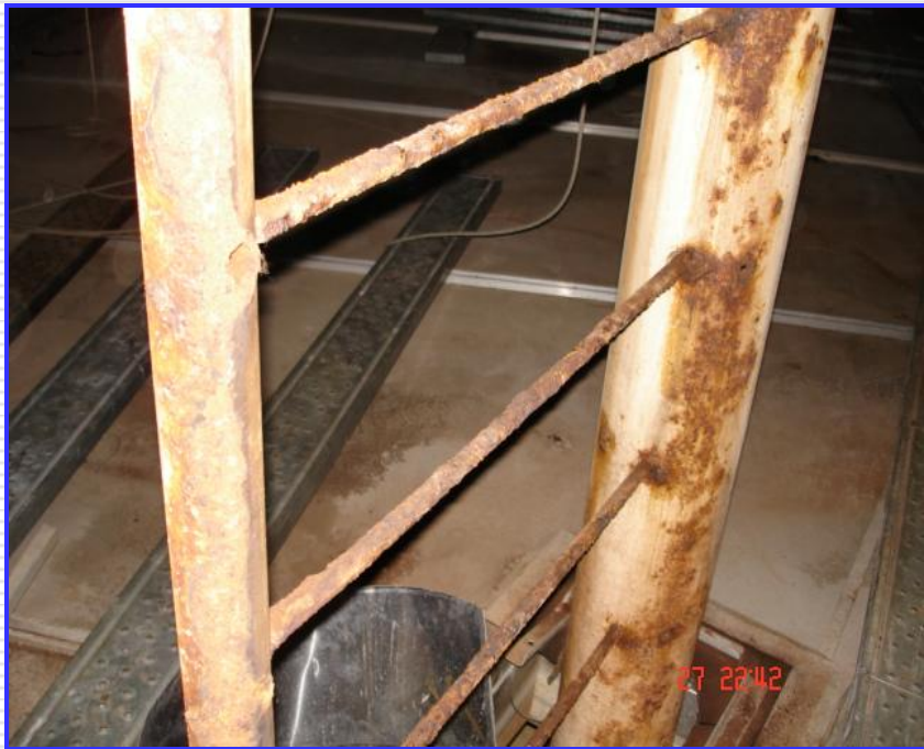
Before Blasting and Painting of Ladder
