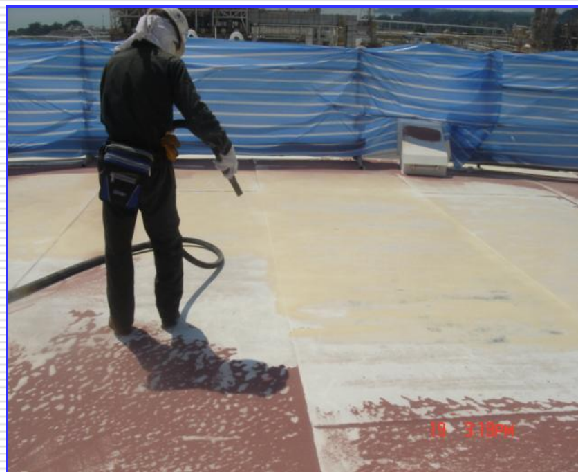
Sweep Blasting of Tank Roof Top
