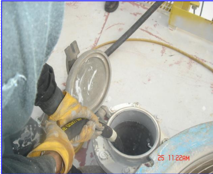
Internal Blasting of Pipelines
